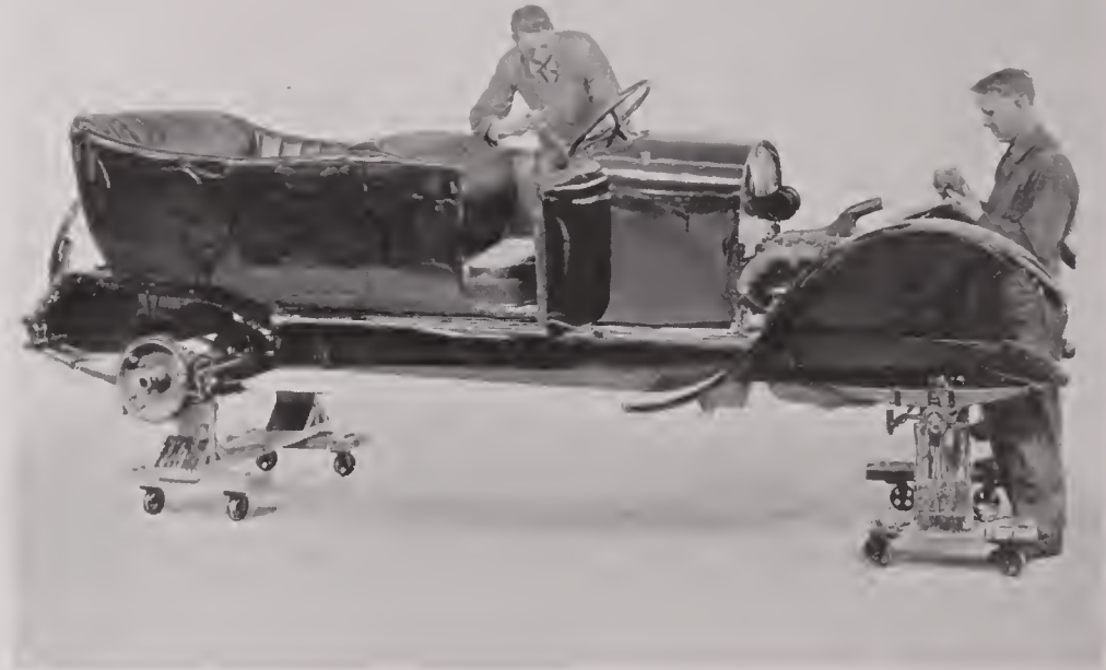
OPERATION NO. 6 Assembling Model 250
